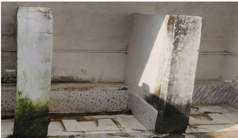
Toilets in a government school
