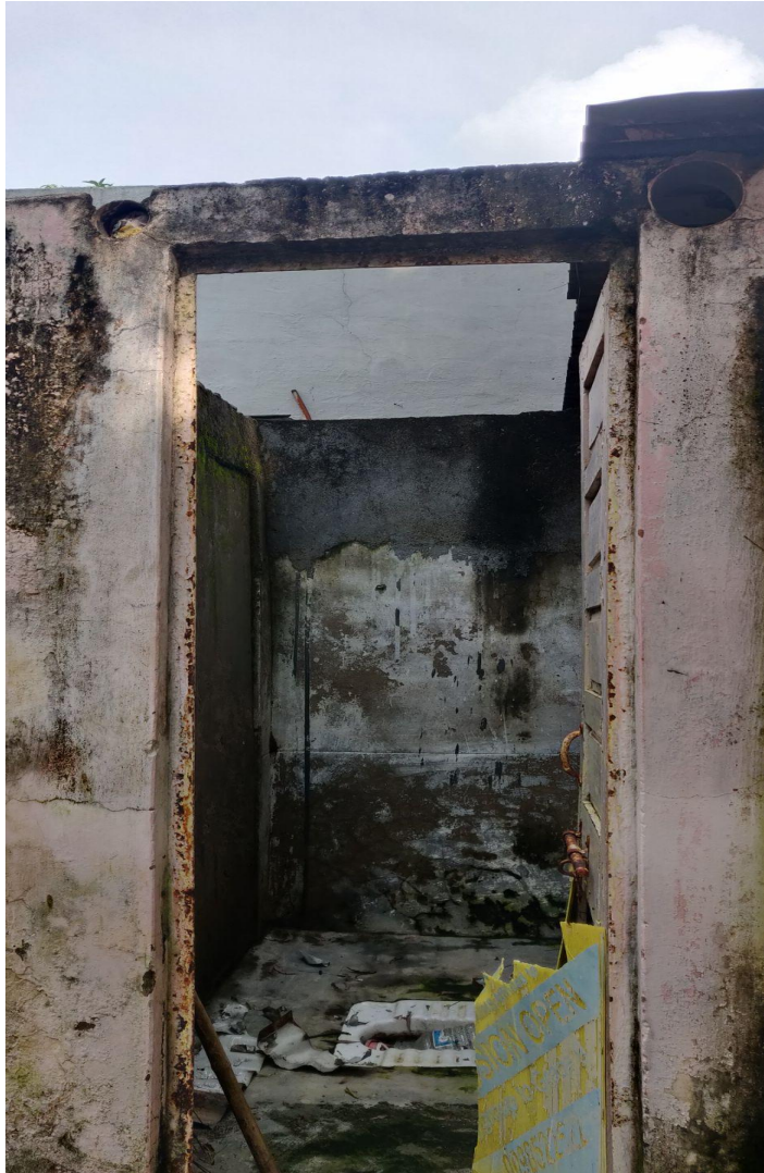
Open roof Toilet in a government school
